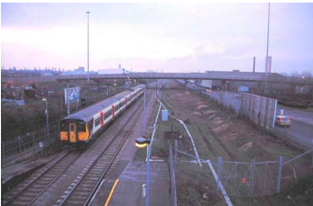
A West Anglia Great Northern service leaving Angel Road, showing the space available for further tracks if required
