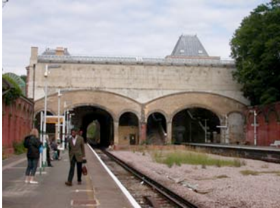
Our offices just show above the trackbed where new platforms for the ELL are to be constructed
