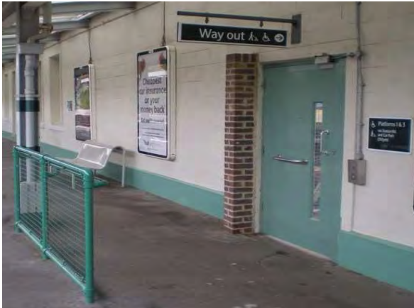
West Croydon Station – to be transferred to TfL
