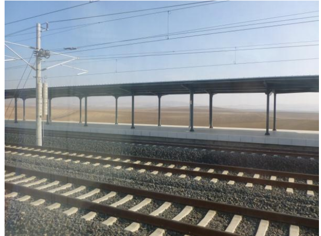
New line works at Polatli
