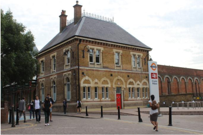
Refurbishment of Crystal Palace station has included the reinstatement of blocked-up windows to our offices
