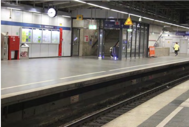
Separate platforms for boarding and alighting (as here at Karlsplatz) clearly help maximise train throughput
