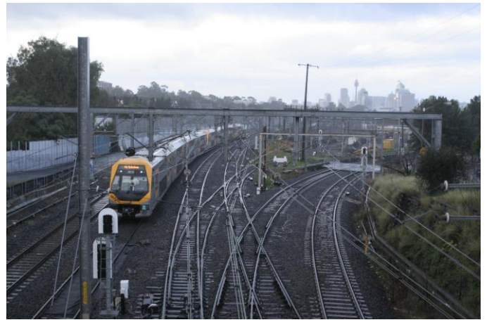
Erskineville Jct: by 2024, a 20tph service will run on the lines to the right, through the CBD, to the 2-platform terminus at Bondi Junction, where operations are going to need to be planned - and managed – very tightly
