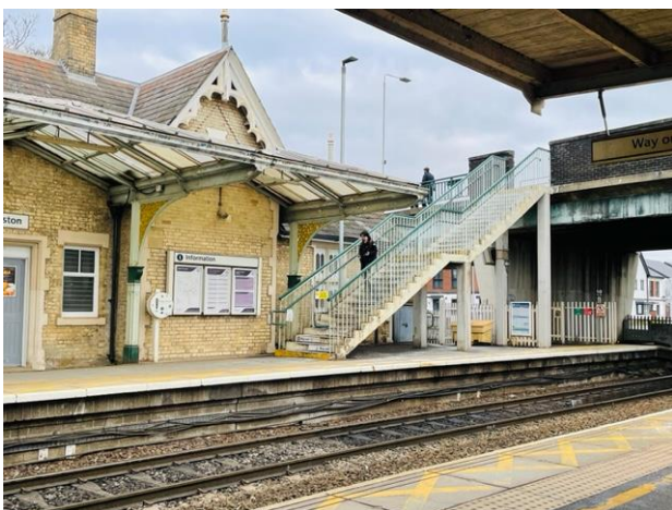
The footbridge at Beeston attracted considerable criticism from local stakeholders
